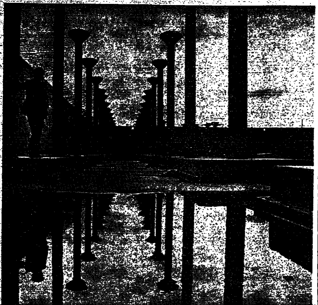
Before the flood: A new 10-million gallon reservoir excavated on the campus of York University by the city waterworks. Its roof will be a university sports area.
